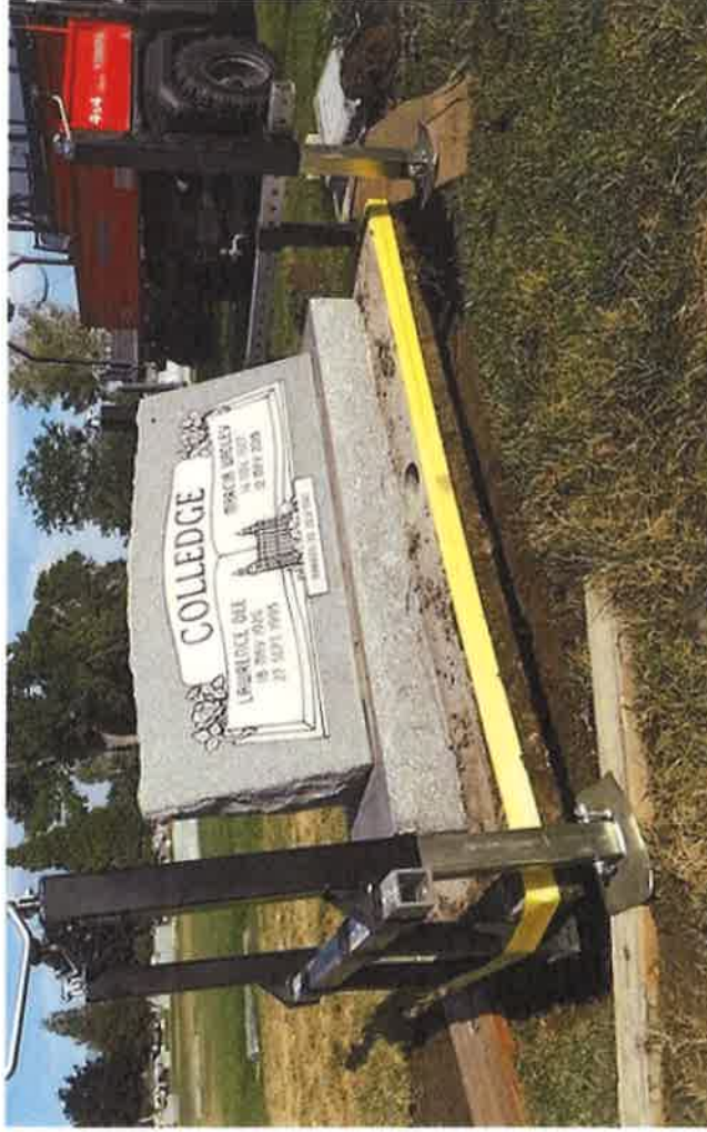
Safe set up with the lift feet and ratchet strap!
