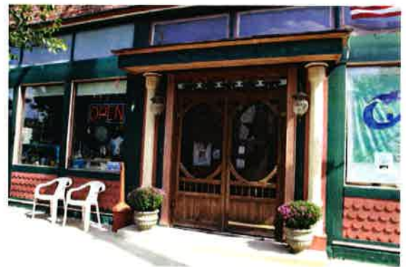
Figure 3.2. Transom windows above the storefront display windows.
